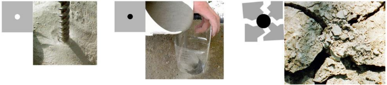
Fig. 9. Phases of the technological process of splitting rock solids with the use of expanding materials [22]
