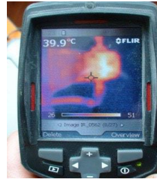
Fig. 26. Proper working pump
