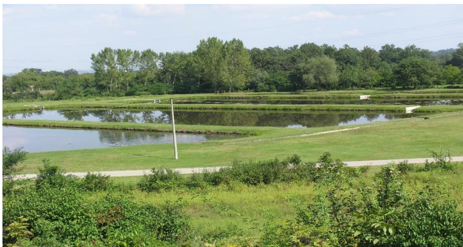
Fig.5. Reclaimed area of the settling tank
