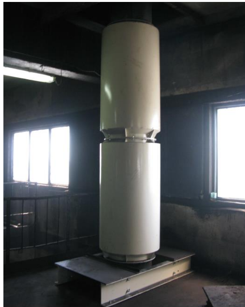
Fig. 5. View of noise silencer of TG type operated in the dust control installation at the coal mechanical preparation plant [9]
