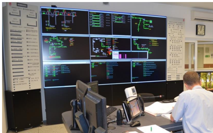
Fig. 4. Tauron's control room [7]
