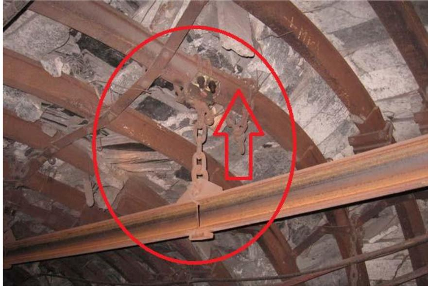
**Fig. 1.** Mechanical failure due to dynamic loads and local deformation of the roof
